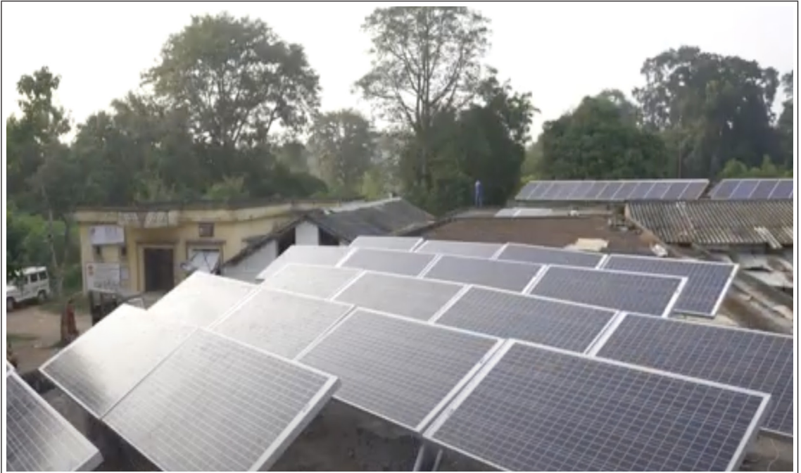
Figure 22 : A 10kWp solar PV Power Plant installed at Nav Jivan Hospital (2017)
