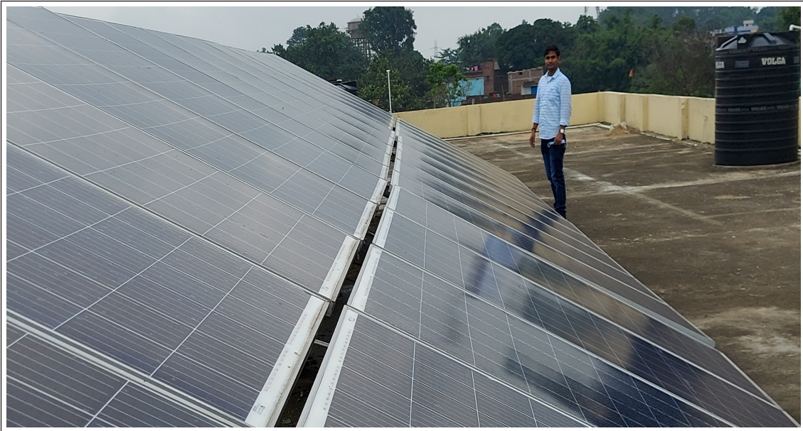
Figure 19. A 10 kWp Solar PV Power Plant installed at Getalsud PHC, Ranchi
