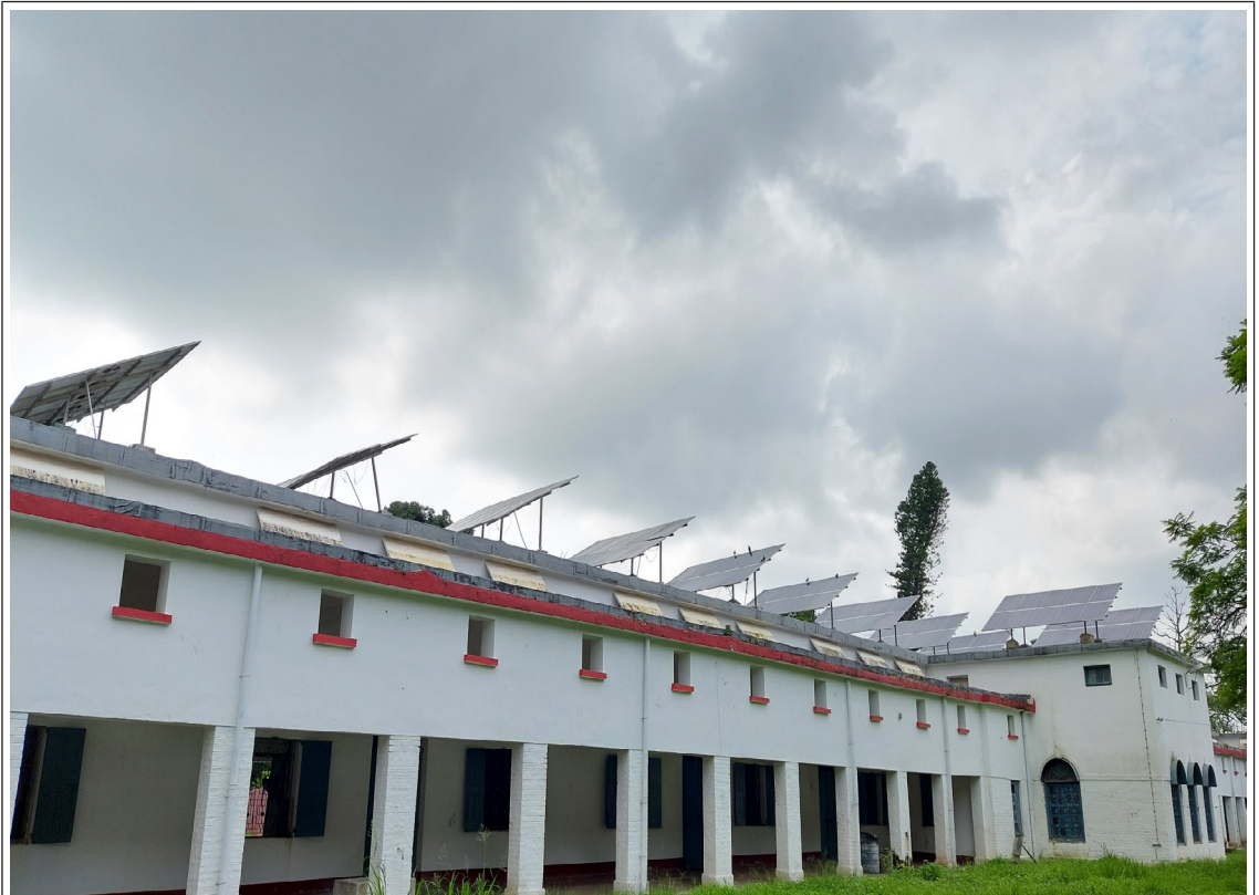
Figure 20. A 50 kWp Solar PV Power Plant installed at female ward of RINPAS, Ranchi
