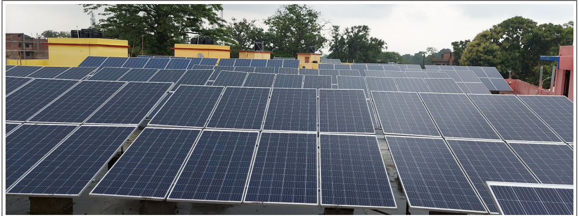
Figure 18. A 50 kWp Solar PV Power Plant installed at Angada CHC, Ranchi
