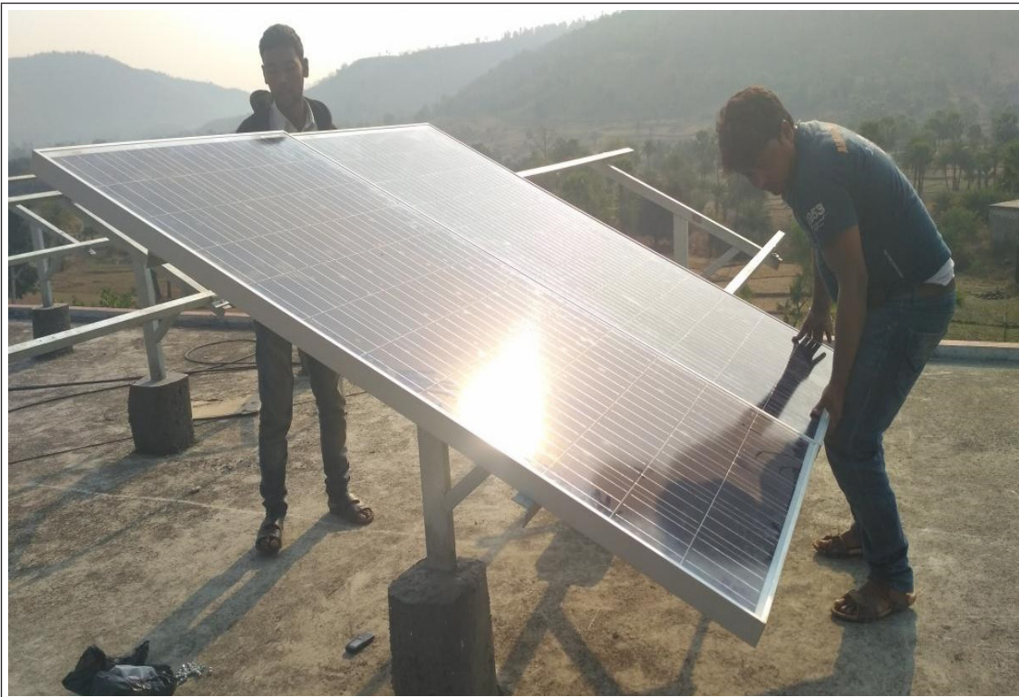
Figure 21 : Installation of a 15kWp solar PV system on the roof of a hospital (2017)
